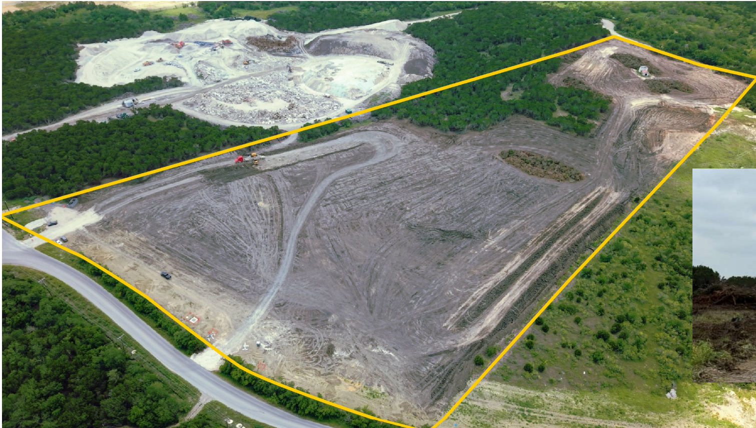
Soils excavation and haul-off underway
