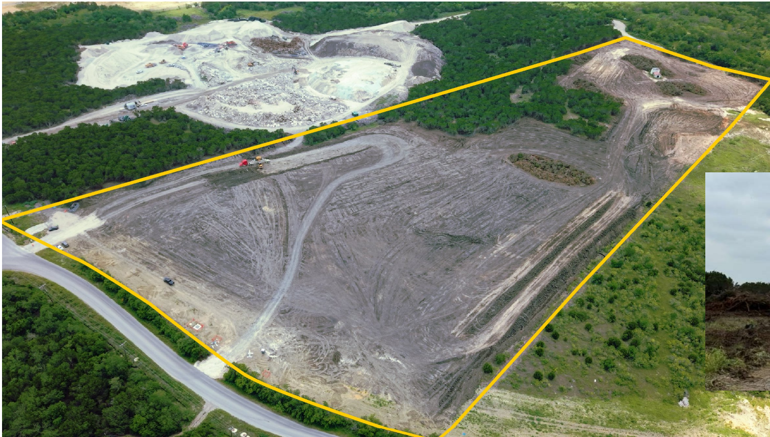
Soils excavation and haul-off underway
